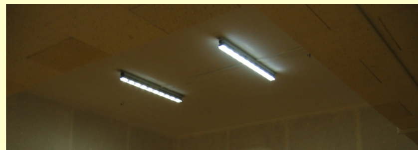
Elevator hall of administrative building of the Neurosurgical Institute
